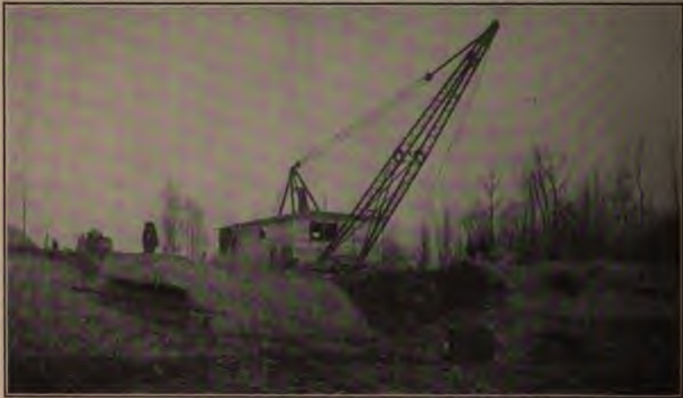
Drag-line Excavator with Steel-framed Boom.
